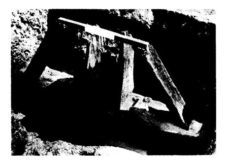
Fig.71 Hammer hurst at Chingley forge (TQ 682335). This construction, the base a re-used timber, related to the earlier of the seventeenth-century hammers, and was covered by working debris after the hammer and hammer-wheel were repositioned (scale: 3ft).
